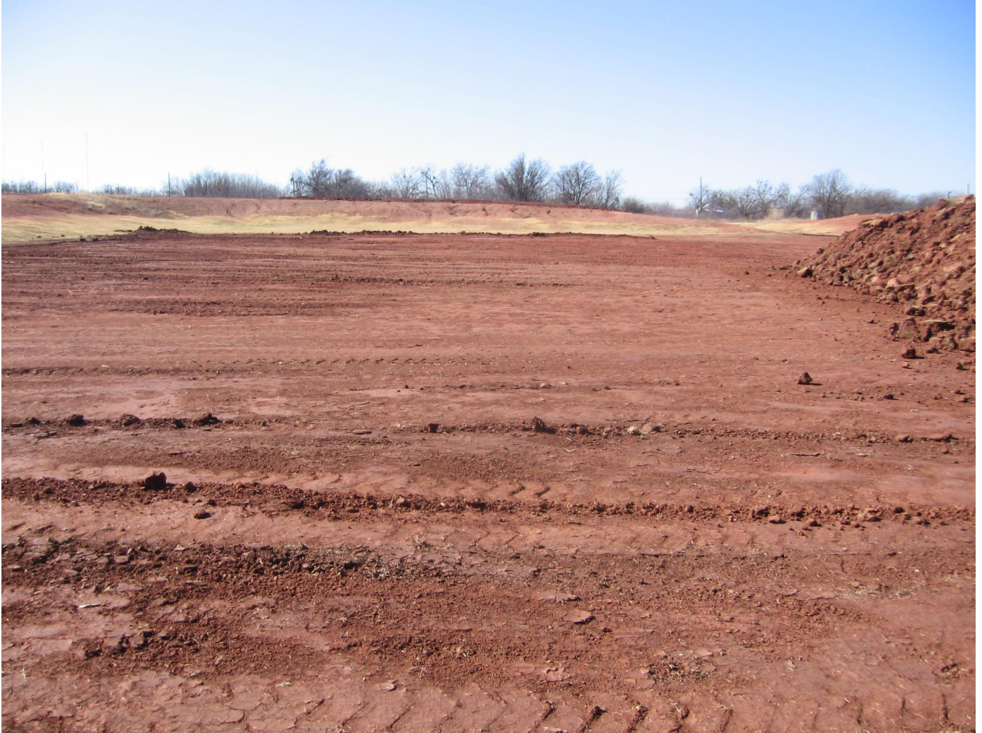
Graded detention pond ready for additional cuts.
