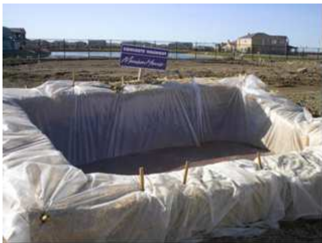
An example of a self-installed concrete washout structure.
