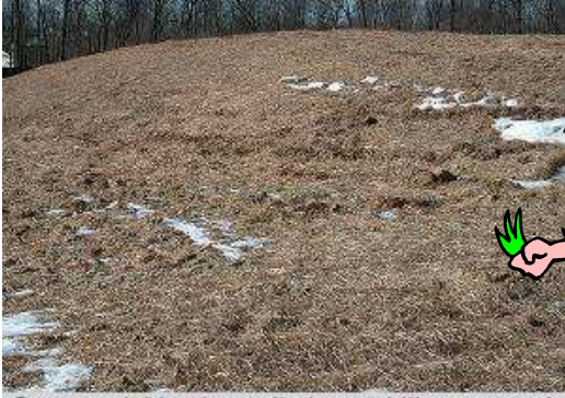
Grass mulching is applied to stabilize exposed soils and to reduce stormwater runoff velocity
