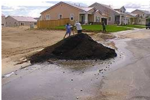
Unprotected stockpiles can cause sediment to wash down the street.
